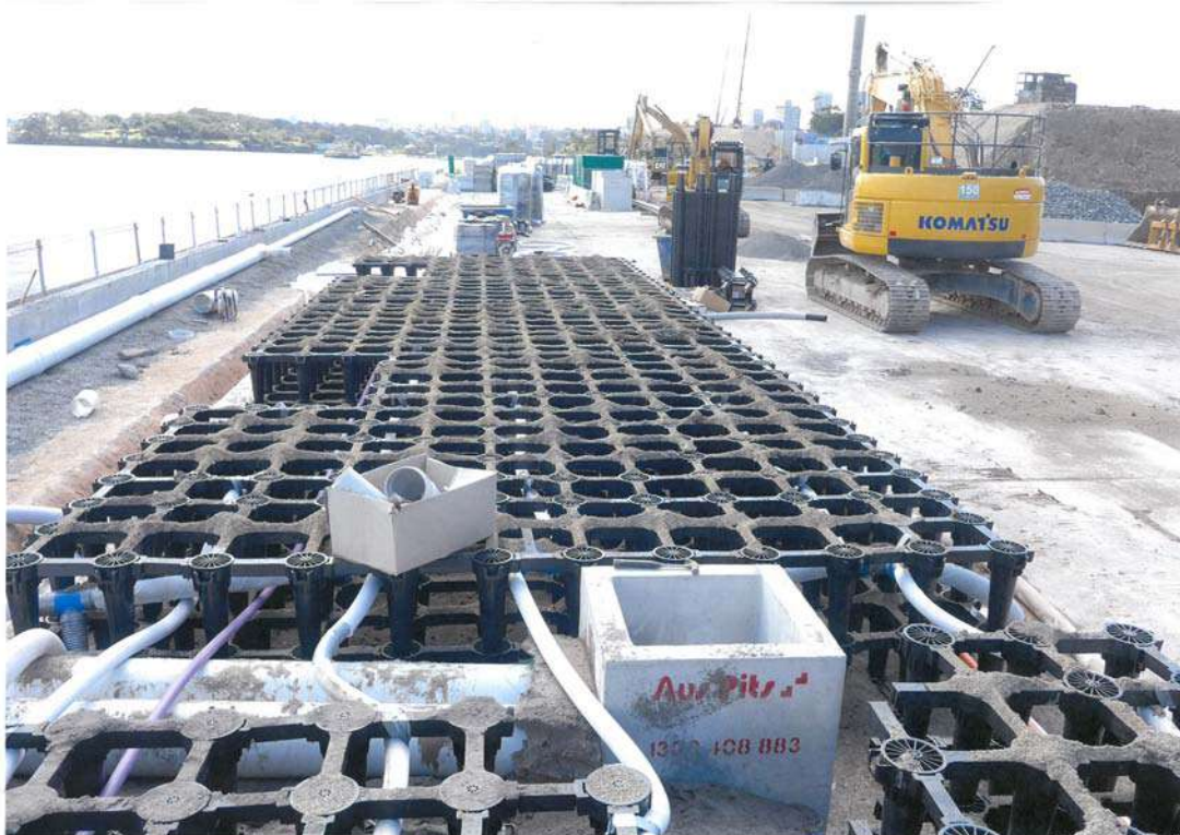
Figure 4.8 –Numerous methods are now available of integrating trees and the necessary soil volumes within urban environments while still allowing pavements and roads to continue successfully above. The above illustrates the proprietary system Strata Vault by Citygreen being used at Barangaroo Sydney.
