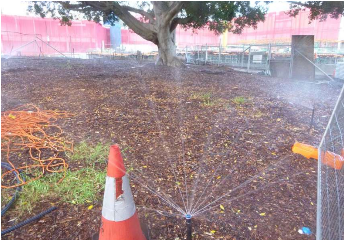
Figure 5.2 – Example of a temporary irrigation system provided to trees during construction periods. This can be a very valuable way of ensuring tree health and vitality is maintained and also promote new fibrous root growth closer to the trees. (Photo: Arterra)
